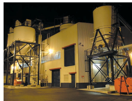
Thermal Drying facility for Hutt City Council, NZ, 2001.
